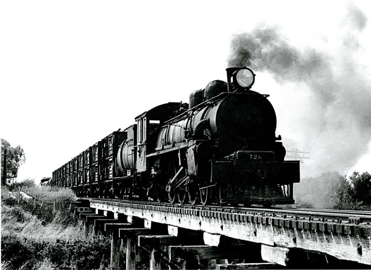
LEFT: A substantial, bridge crossed the Waimea Stream, north of Mandeville. It was the setting for this scene as AB 726 worked a southbound N o 576 Goods to Gore in February 1968. The bridge, N o 4 on the branch, was 207 feet (63.1m) long.
